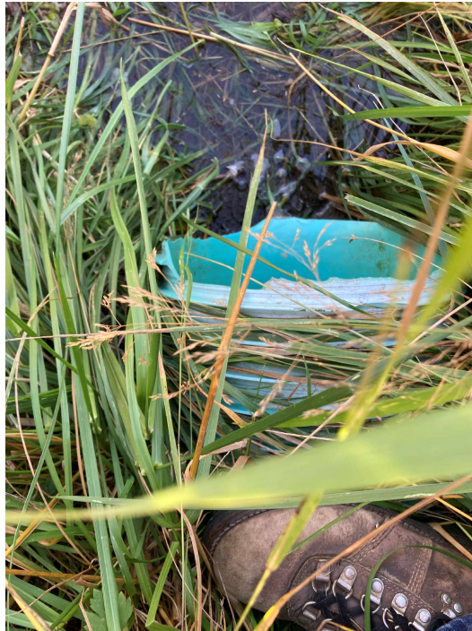
Photo 2. View looking at the culvert at the downslope edge of the dugout, located 3 m above the water level, with water draining from the roadside ditch into the dugout. September 21, 2022.
